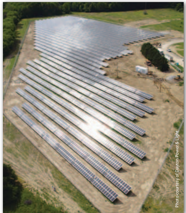
Aerial view of Dayton Power & Light's 1.1-megawatt solar array in Washington Township, Montgomery County, Ohio.
